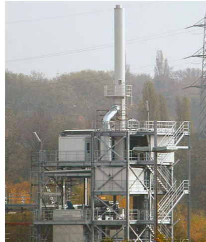
Incineration plant for waste gases containing silane
