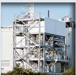
Combustion plants for the disposal of exhaust air, waste gases and liquid media
